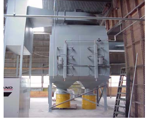
DUST COLLECTOR PULSE CONTROLS
