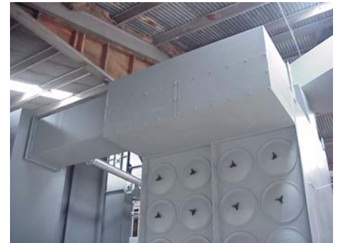
ABRASIVE INLET DUCT
