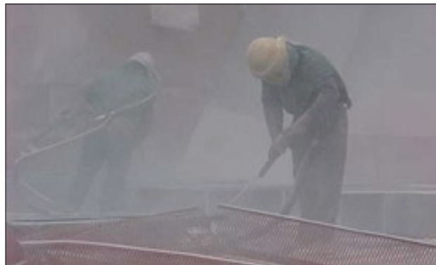
Abrasive blasting creates high levels of dust. Photo courtesy of NIOSH © NIOSH & Associates
