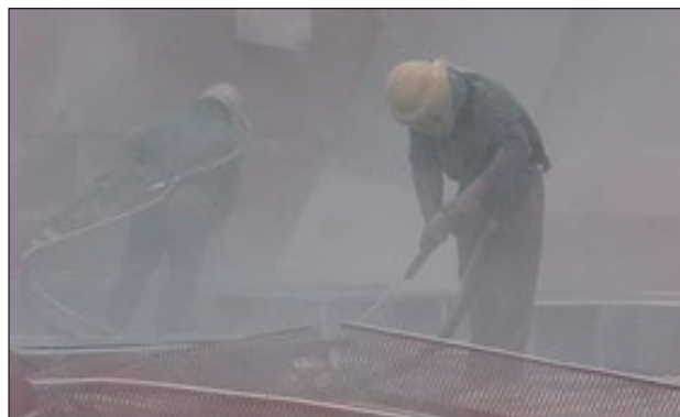
Abrasive blasting creates high levels of dust. Photo courtesy of NIOSH © NIOSH & Associates
