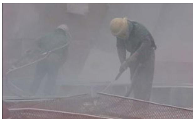
Abrasive blasting creates high levels of dust. Photo courtesy of NIOSH-Hess Manufacturing, Inc.
