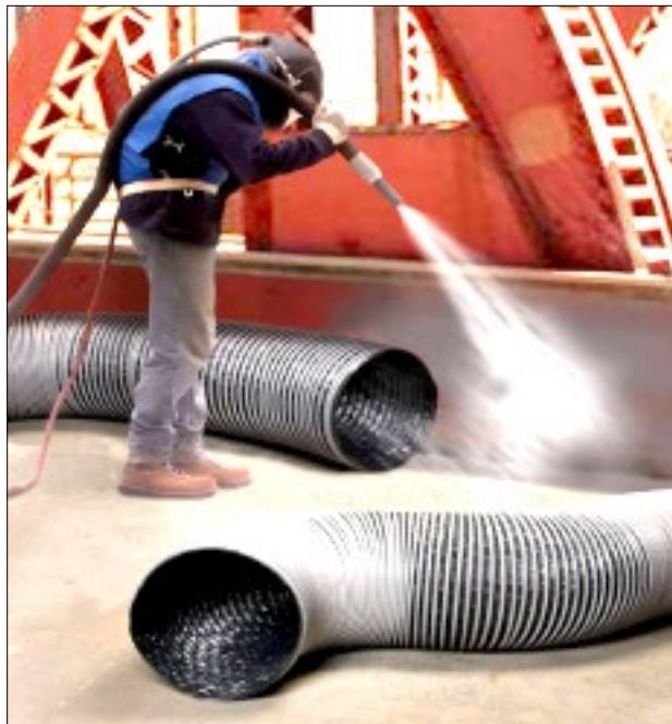
Abrasives blasting using a dust collection system with multiple exhaust ducts. (Photo courtesy of Flexaust, Inc. This equipment is shown for illustrative purposes only and is not intended as an endorsement by OSHA of this company, its products or services.)
